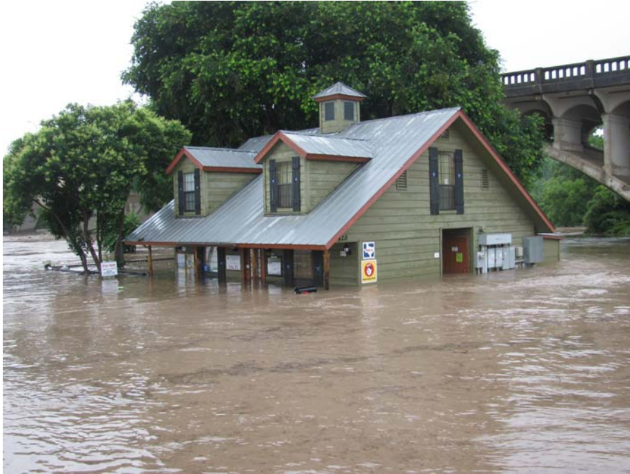
Photo 1, RV Park underneath I-35 bridge at the Guadalupe River
