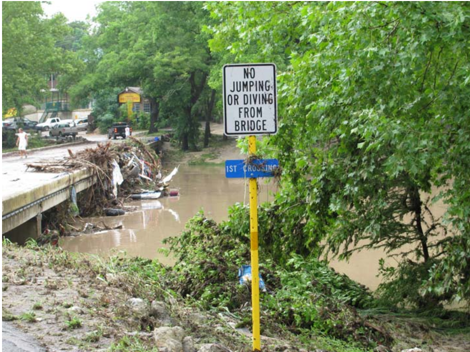
Photo 8, Bridge Crossing #1, River Road at the Guadalupe River
