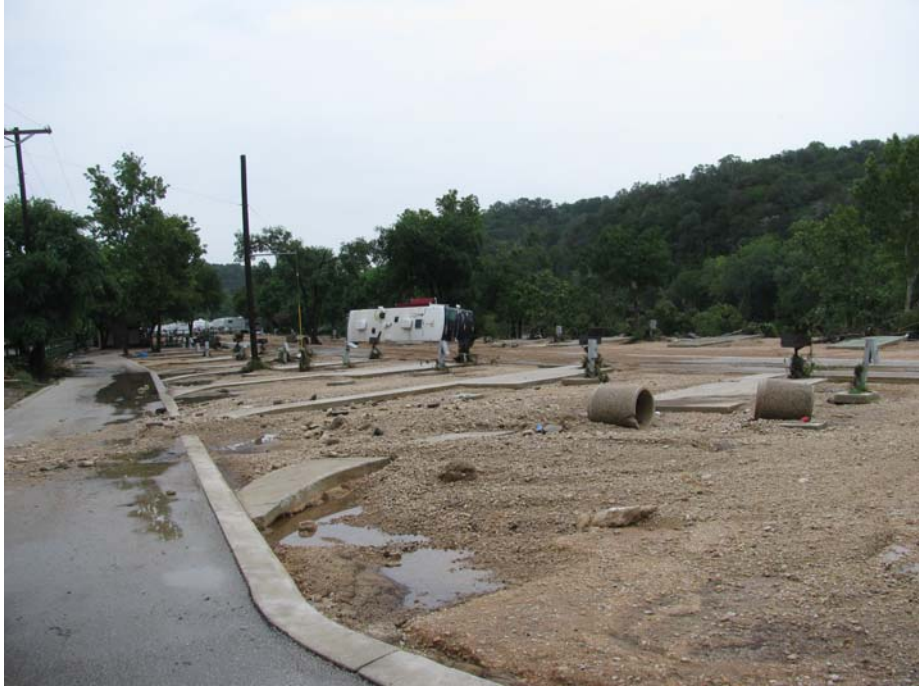
Photo 7, Remnants of a campground along River Road downstream from Crossing #1
