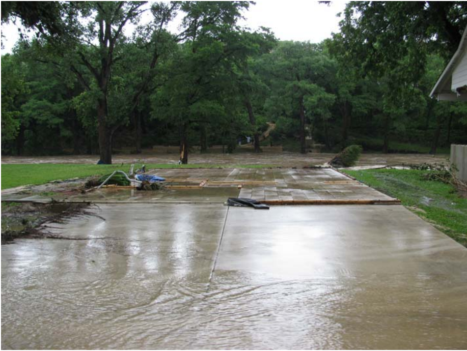
Photo 4, Home swept off it's foundation in Gruene
