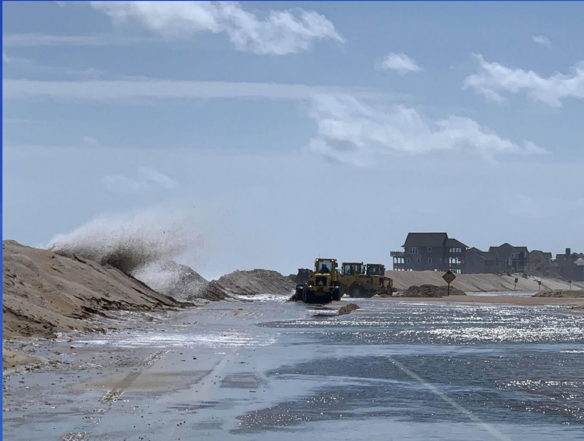
Powerful swell flies over weakened dunes along Highway 12 on the Outer Banks of North Carolina while NCDOT road crews attempt to rebuild.
