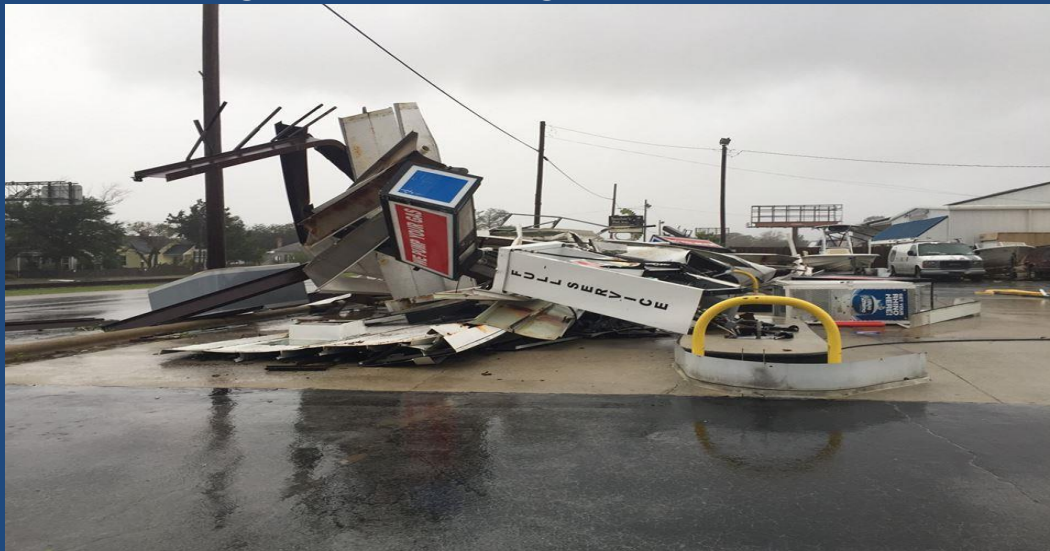
Damage in Morehead City following Hurricane Florence, September 14, 2018.
