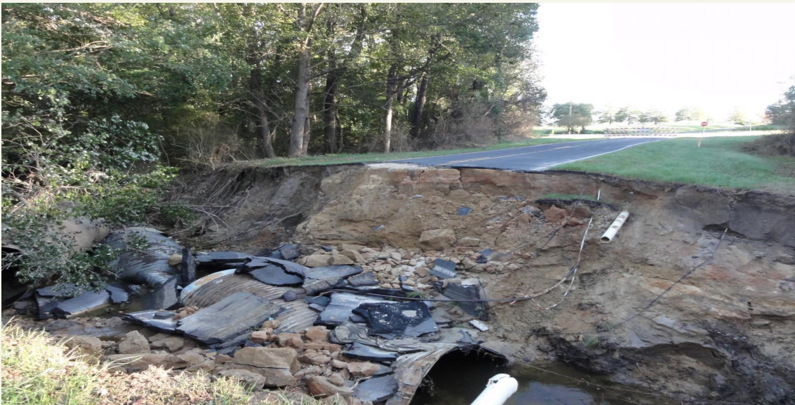
Washed out road in Greene County. This is why we urge folks when you see water covered roads to Turn Around, Don't Drown!
