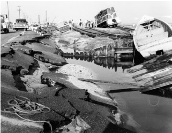
Damage to the Beaufort-Morehead City Causeway
