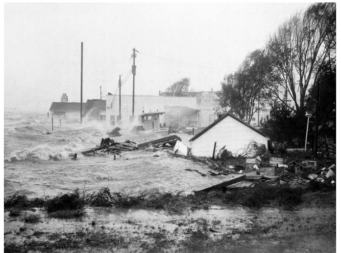
Severe Surge Flooding in Morehead City
