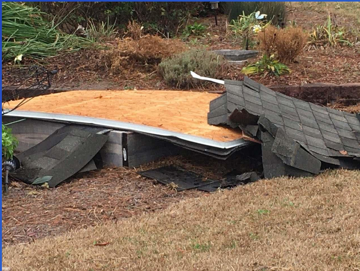
Roofing damage from strong winds near Pollocksville, NC late on December 24, 2020. Photo credit: Ivey Riggs
