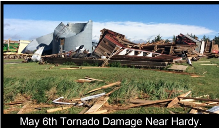
May 6th Tornado Damage Near Hardy.
