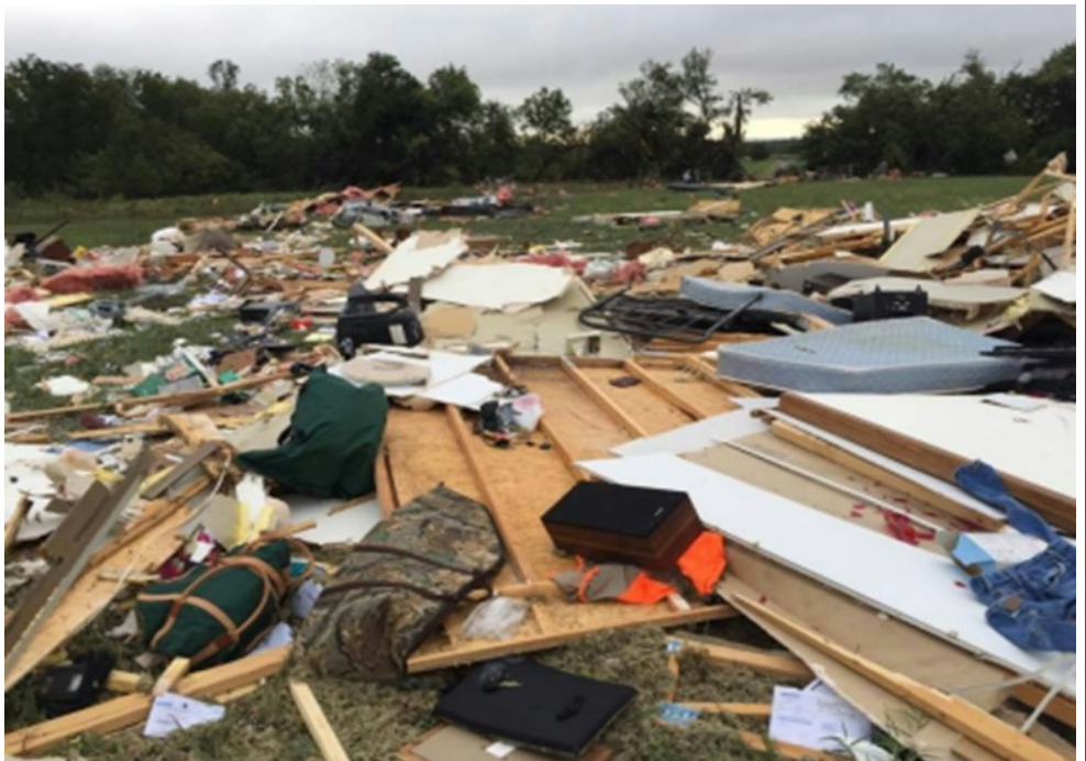
Damage from Tornado near Hillsdale Lake (Miami County, KS)
