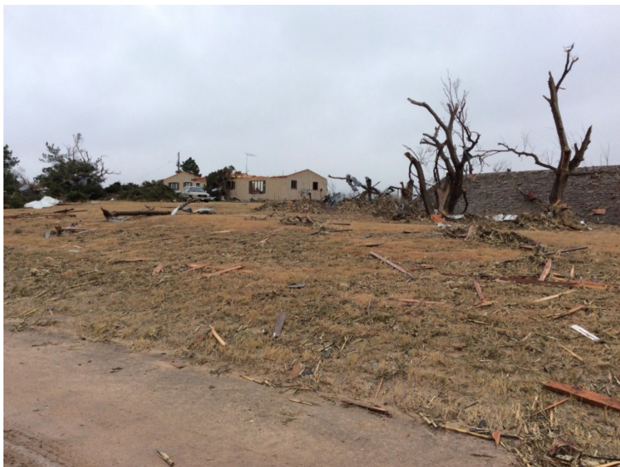
Damage to hog farm west of Kismet on November 16th, 2015. EF3 damage
