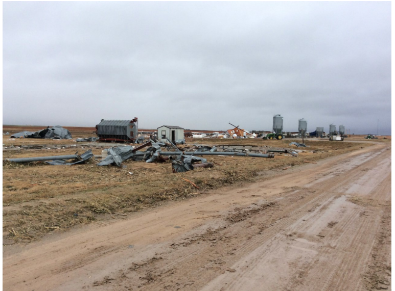
Damage to hog farm west of Kismet on November 16th, 2015.
