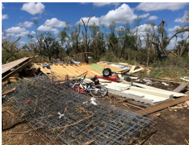
A flattened storage shed after the passage of a tornado near Formoso, KS on May 6. NWS storm survey photo.
