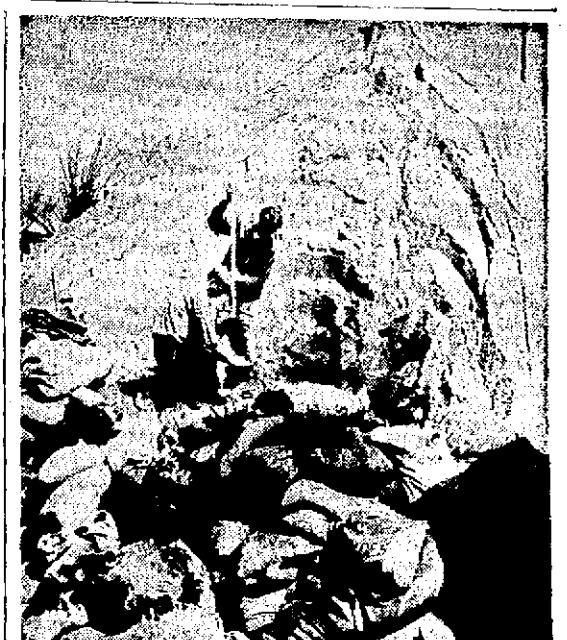
FILLING THE BAGS . . . Filling bags from a mountainous pile of sand at a street department stockpile are these two workers, part of a crew which began work Thursday. Bags will be used to line exposed sides of protective levees around the city. Most of the 240,000 bags now on order will be in Winona by Monday, city officials learned today. (Daily News photo)
