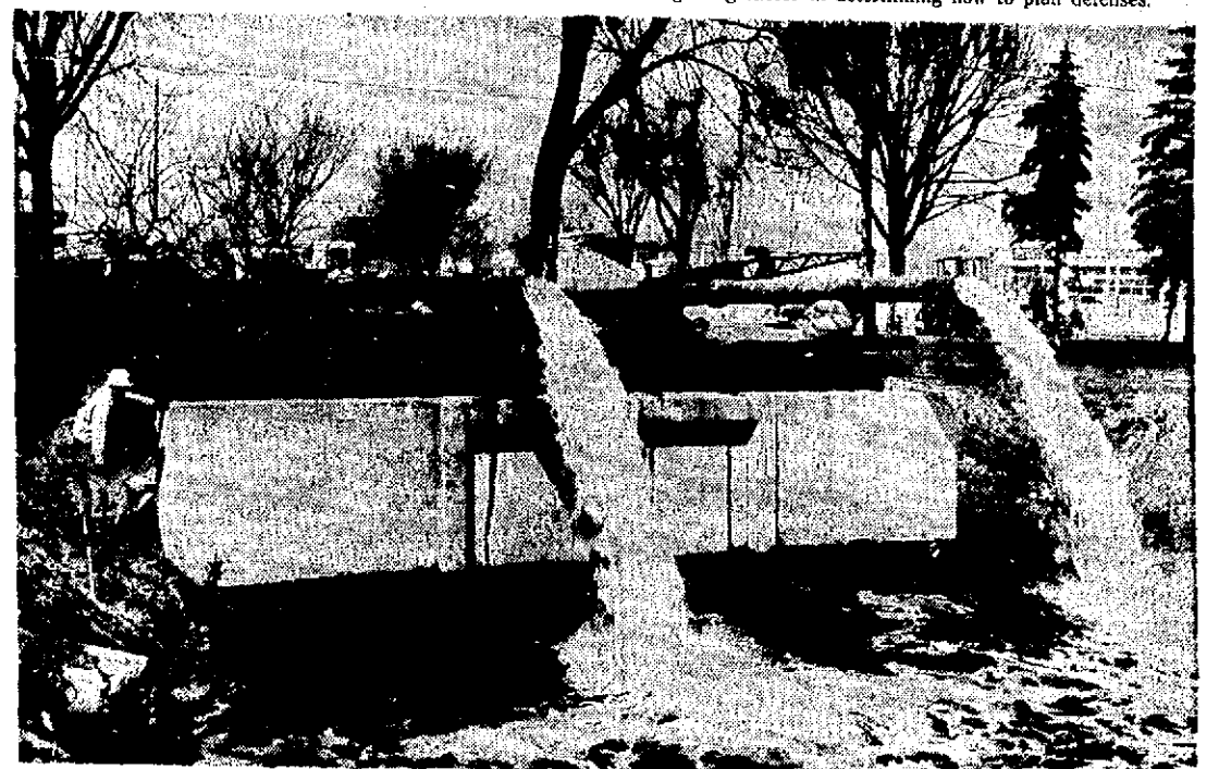
LAKE PUMPS . . . Dumping 10,000 gallons a minute into the Lake Winona outlet ditch are two pumps, due to be reinforced today by two more of the same size. Pumping was going on around the clock as engineers tried to hold rising lake levels in check. Heavy runoff from Gilmore
