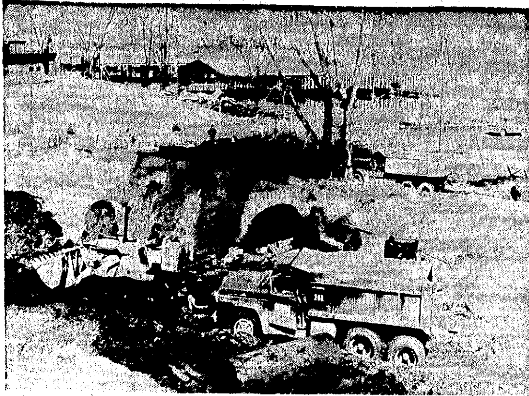
FILTER SUPPLY CORP. . . . Crews have been working two days to build a dike around this Miller industry at 580 E. 2nd St. Cooperating in the effort is Winona Industries, Inc., which is situated on adjacent land. Whittaker Marine & Manufacturing is in the background. (Daily News photos)
