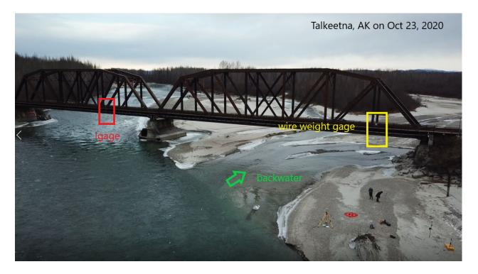
Figure 11: shows a photo from an APRFC UAS mission at the railroad bridge at Talkeenta, where flood levels have also recently been adjusted. Historic measurements took place at the wire weight gage, which has been impacted by sediment buildup. This photo was taken during the extreme low flow conditions of late October.
