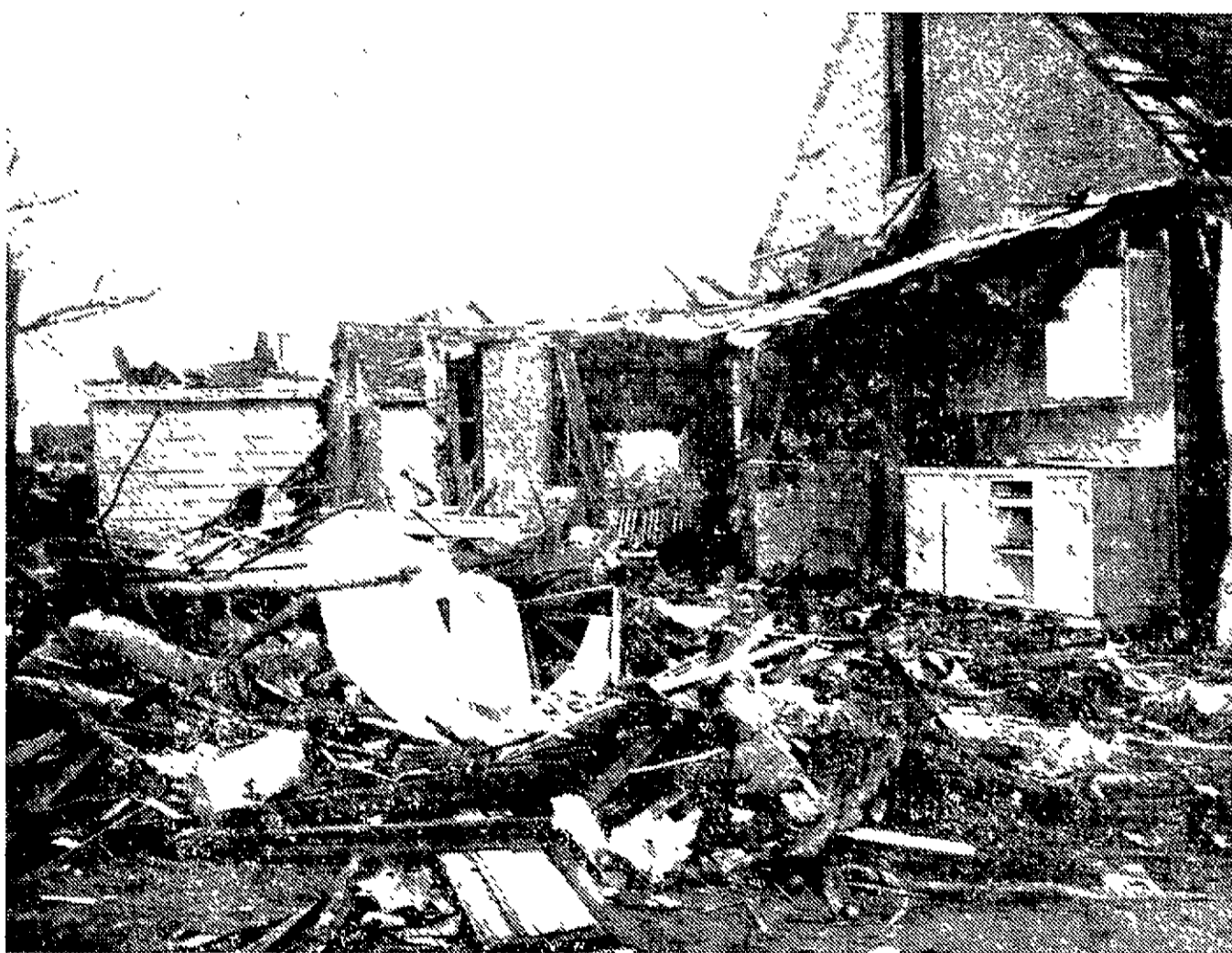
Even those houses still standing were so badly damaged that literally scores of them are being tagged as unsafe and will have to be torn down completely before rebuilding operations can get under way.
